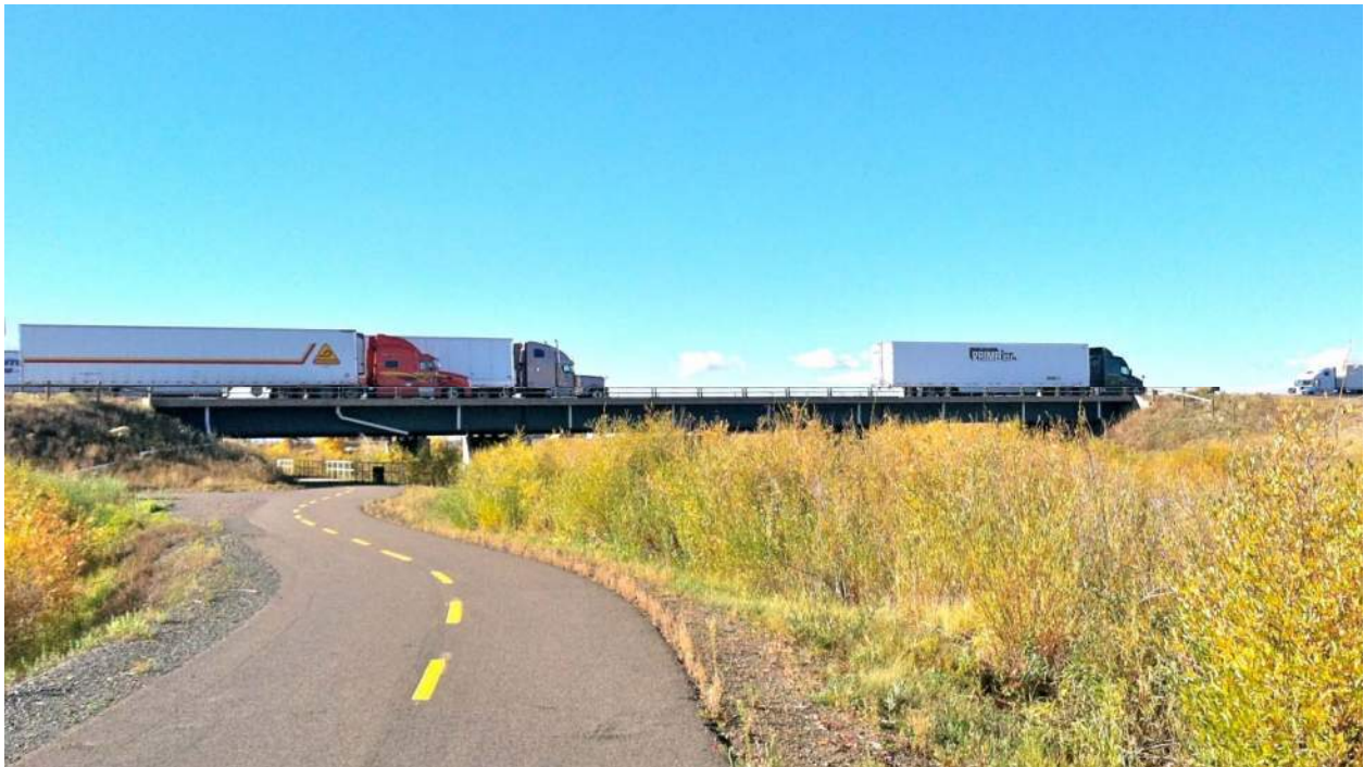
Figure 1: Laramie River Bridge
