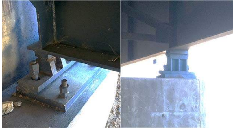
Figure 4: Expansion Bearings at Abutment Two (left) and Pier Two (right)
