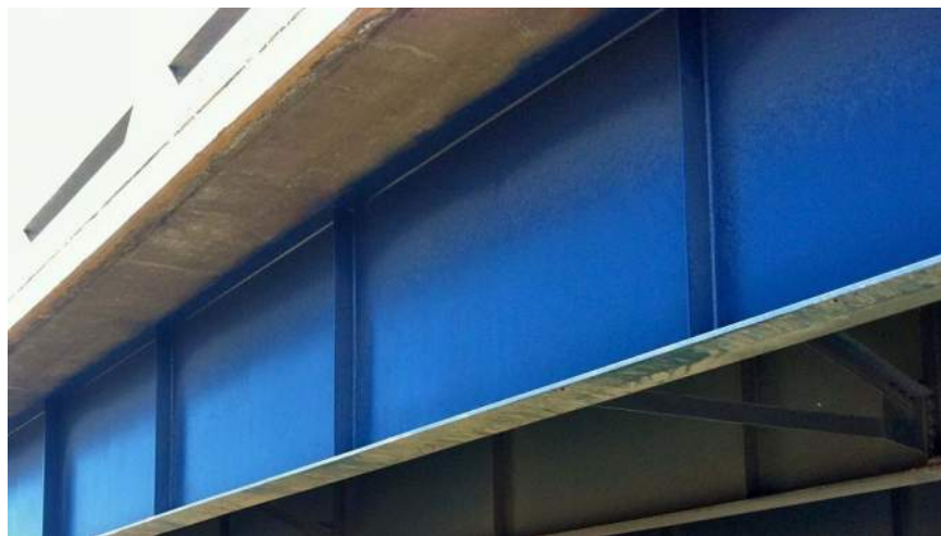
Figure 3: Exterior South Girder
