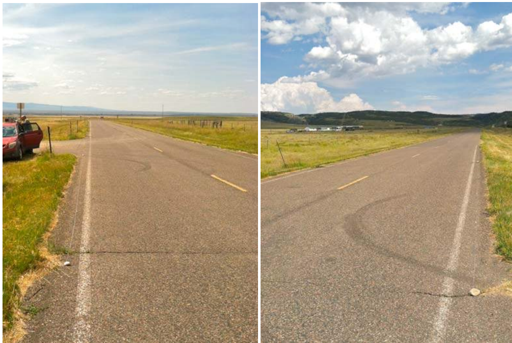
Figure 43: Testing Location on Highway 17 with the West (left) and East (right) Views
