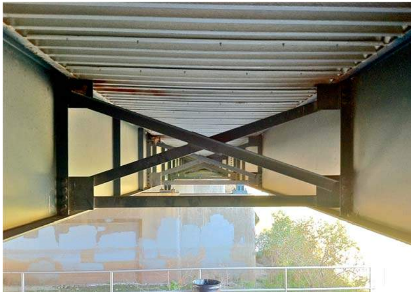
Figure 5: Cross Frames Located in Spans One, Two, and Three and at the Piers
